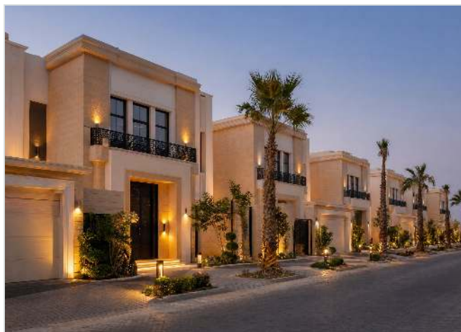
Luxury Villas Development Al-Khomrah Villas, Jeddah
