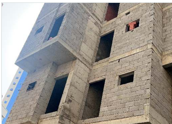
Structural Concrete Frame
