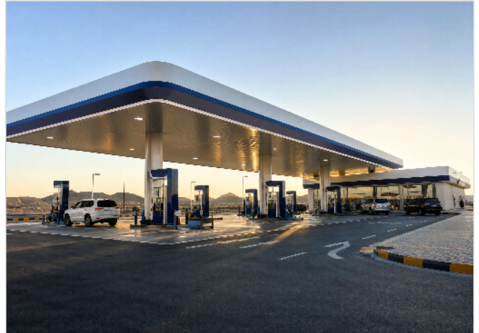
Integrated Station with Service Building Western Region, Saudi Arabia
