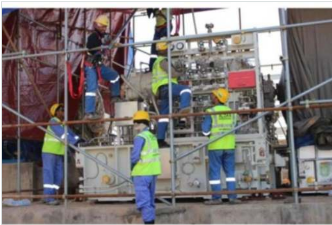
MEP Installation Works NDC Electromechanical Crew
