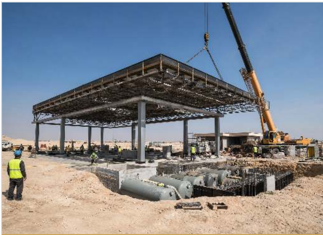
Station Under Construction — Steel Canopy Erection NDC Site Works
