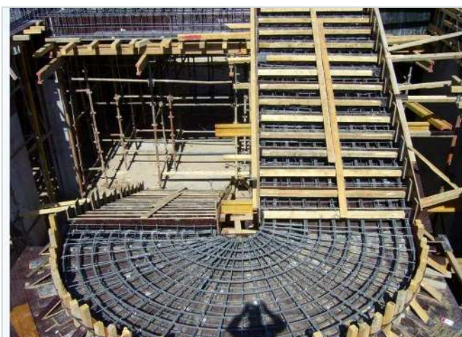
Slab Reinforcement Works
