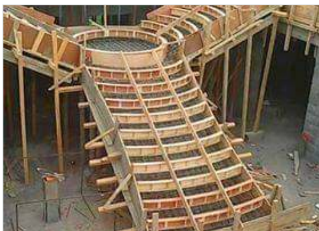
Staircase Formwork & Shoring
